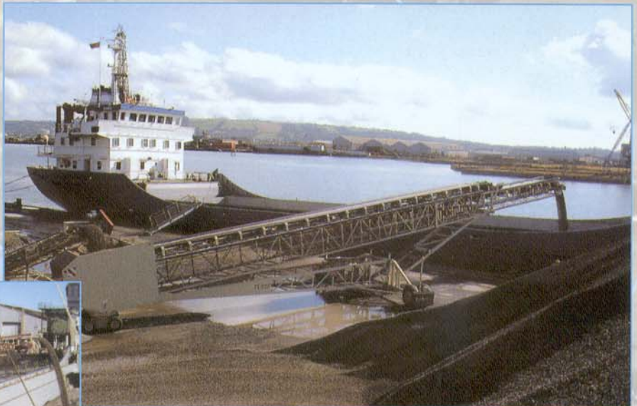
Shiploading Conveyor Control
